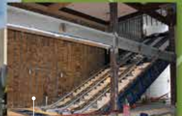
Phase 3 began December 2016 Renovations to existing Boise Centre
