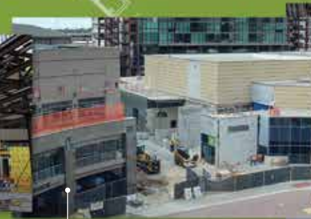
Phase 2 began July 2016 Connecting Concourse
